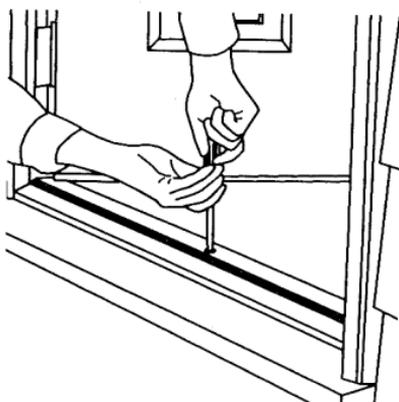
Loosen the anchor screws to allow movement. Then raise or lower the sill. Repeat the process until you are satisfied with the seal. Do not make it too tight or the seal will wear out - too loose and you will have air leaks. When you have a snug fit, tighten the anchor screws with a screwdriver.
