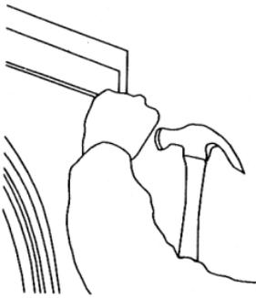
After the door is centered, anchor the door in place. First, nail through the metal door frame on the hinge side in the holes provided. Place a nail in the top hole of the lock side. Then close the door and eye the margin down the side, you may need to tap the frame a little to adjust it.
